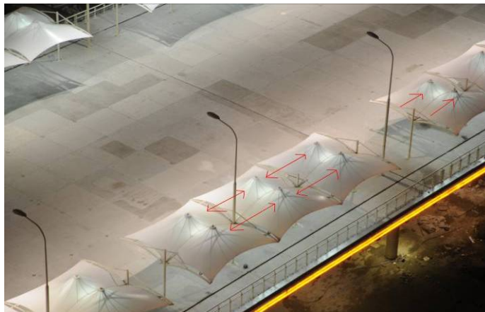
上海世博高架人行步道照明 High Power LED
